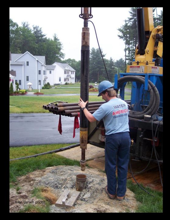
A hydrofracture "packer" about to be lowered into a well
